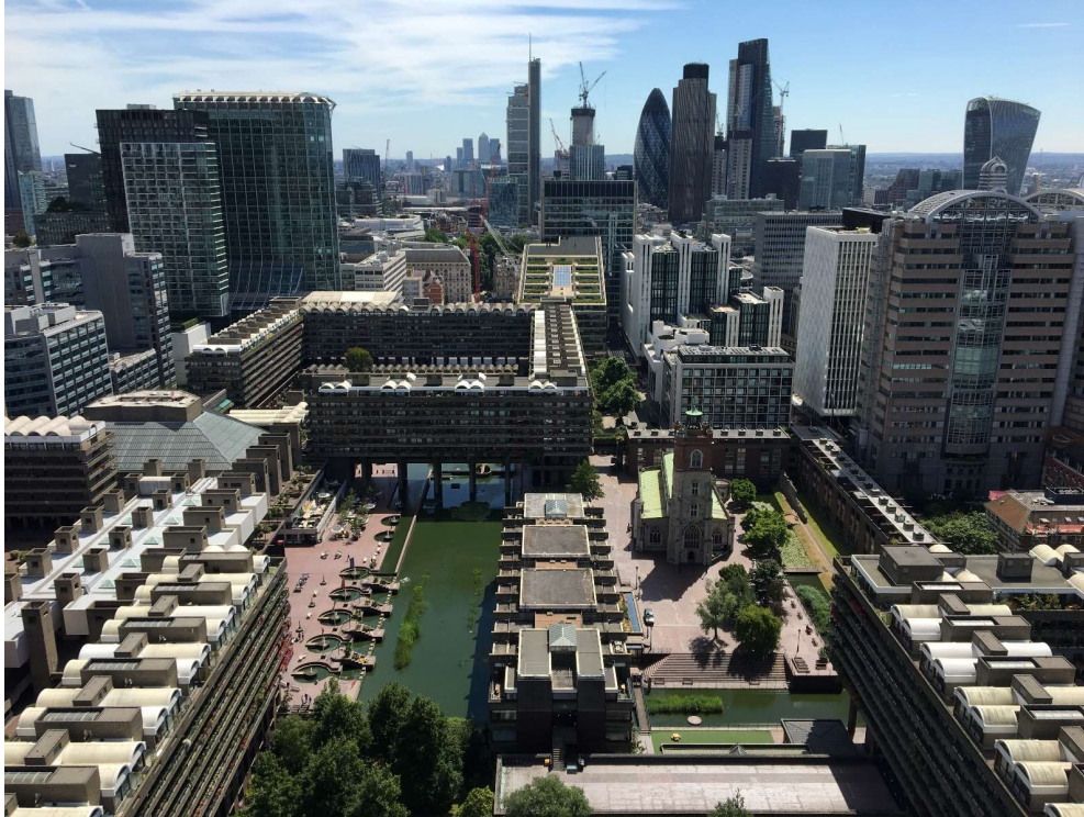
Looking west over the Barbican Estate.
