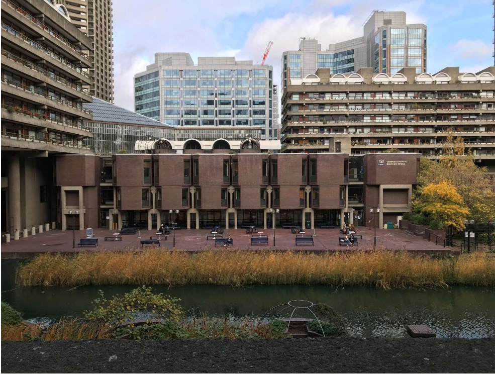
Looking north across the lake to the Guildhall School of Music and Drama, with Gilbert House to the left and Speed House beyond.
